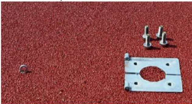
Correctly embedded standard anchor
