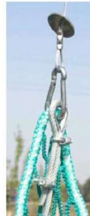
Extreme pillar steel rope fastened to cage net.
